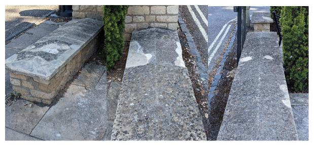
Several areas of coping stone in the lower area of the War Memorial have been damaged as seen in the photographs above. Our approved stonemason has recommended that they be replaced rather than repaired as the damage is extensive – repair work would look unsightly and would not be a long-term solution.
