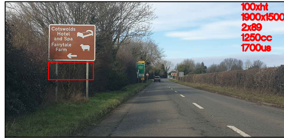
Supply and fit new sign on existing posts under existing sign. (Arrow - text - symbol slightly compressed to achieve 1900mm width).
