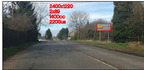
Supply and fit new sign on existing posts on rear of existing. (Arrow - text - symbol slightly compressed to achieve 2400mm width).
