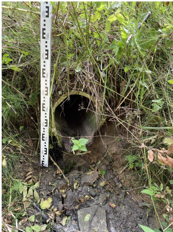
Photograph 10 - Combined sewage outfall at Pool Meadow
