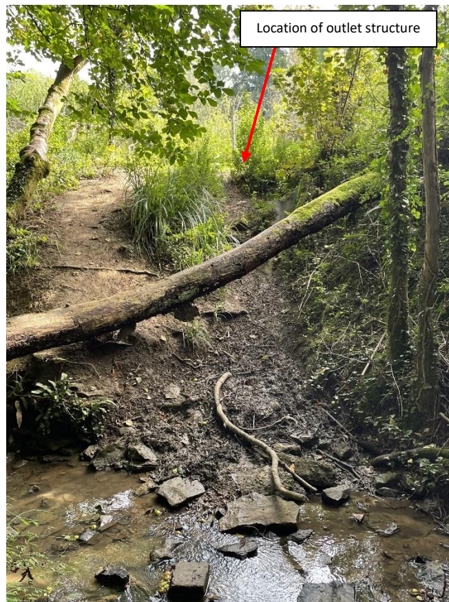
Photograph 8 - location of outlet structure
