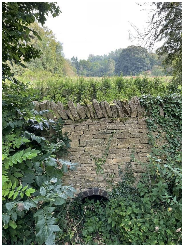
Photograph 4 - Partially collapsed culvert under the track, with upstream meadow in the background
